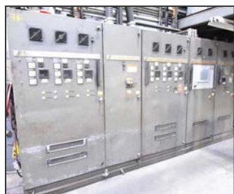
View of ALLEN BRADLEY furnace controls
