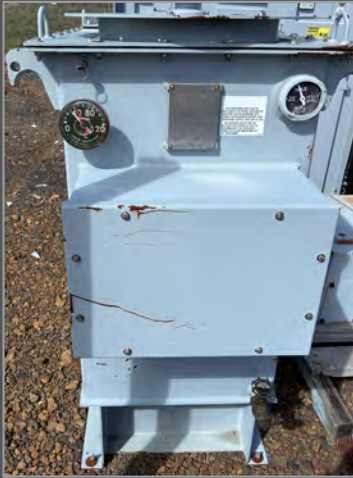
STEIN INDUSTRIES transformer-rectifier power unit
