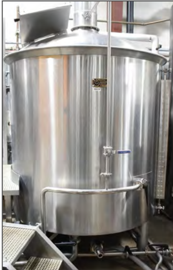
SPECIFIC MECHANICAL SYSTEMS 600 gal. capacity SS jacketed brew kettle
