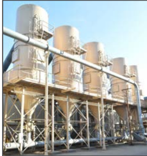
Partial view of dust collection system
