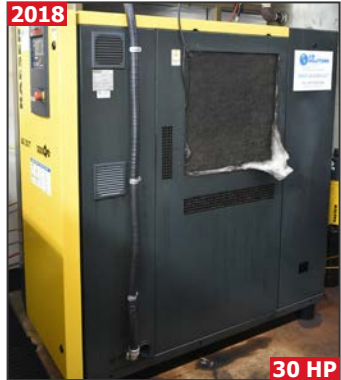
KAESER AS30T rotary screw air compressor
