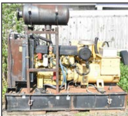
CATERPILLAR D150-8 205KW generator set
