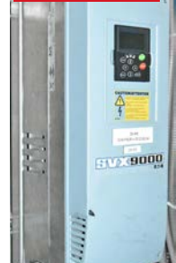
Partial view of EATON SVX VFDs
