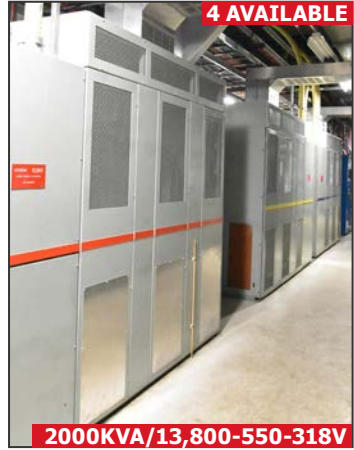
Partial view of POLYGON dry type transformers
