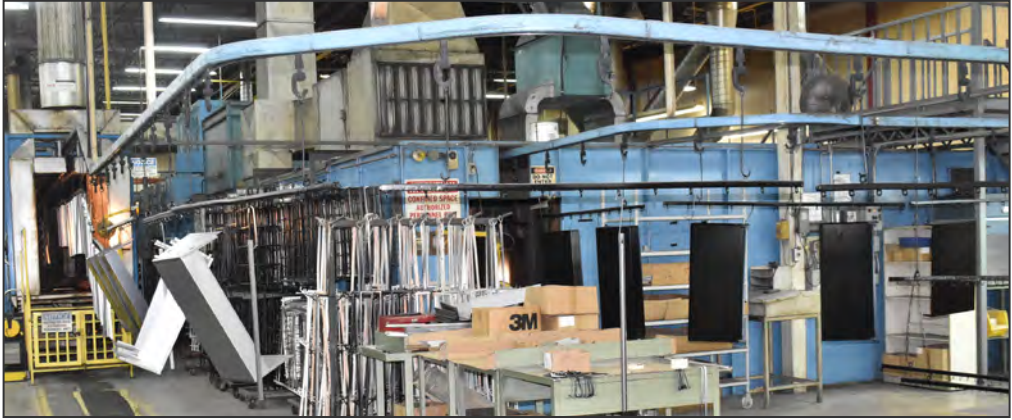
View of 3-stage stainless steel wash system
