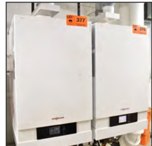
VISSMANN VITODENS natural gas-fired condensing boilers
