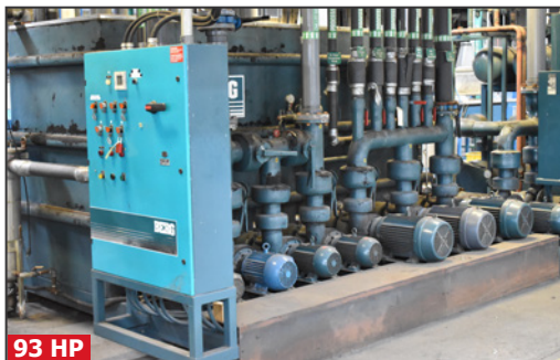
93 HP BERG CT-1146 skid mounted chiller pump set
