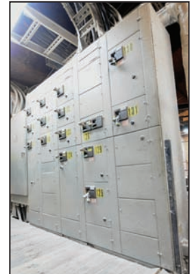
Electrical switchgear
