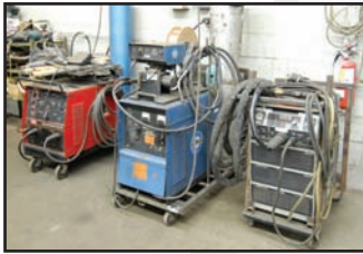
view of welders
